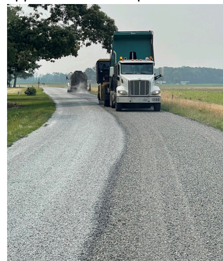
Pictured Above: Chip Seal Paving in Division 4.
